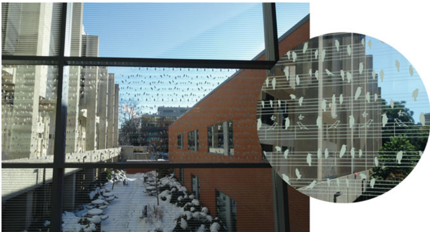
Fig. 3 “Bird’s Eye View” winning design installed at the Tuttleman-Paley connector bridge
